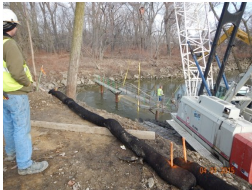
Collector being lowered into river
