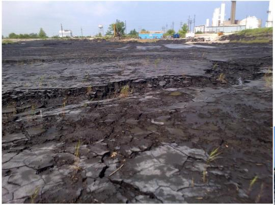
Binder added dry 20% by weight. UCS goals range from 1,000 psf to 1,500 psf (0.05 to 0.07 MPa. Unconsolidated shear strength goal of 1,250 psf (0.08 Mpa) Mixing depths variable - 5 - 20 ft.
