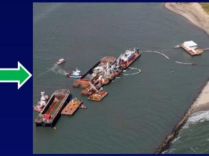
Hydraulic Unloading of Scow Barge and Pump to Fill Area
