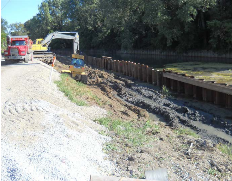
Excavation work in the west side of Zone 1
