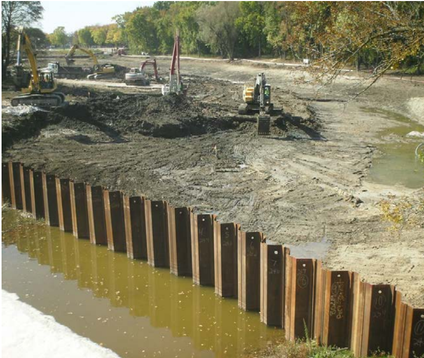
Excavation of northern end of Zone 2a (10/8/11)
