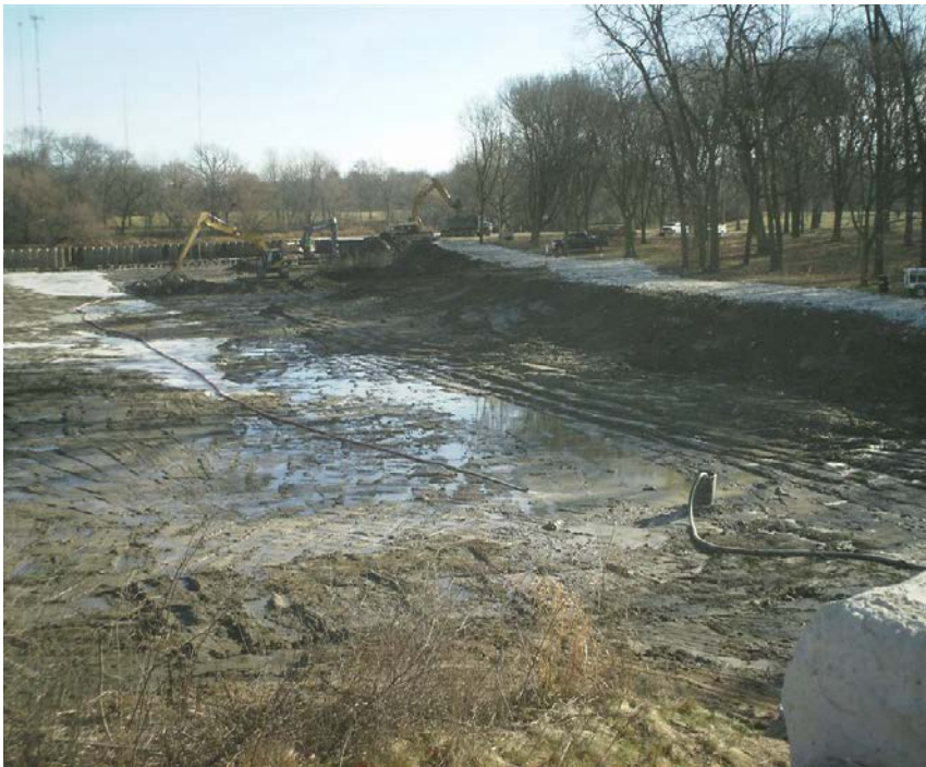
Excavation of sediments and dewatering activities in Zone 3A (1/5/2012)
