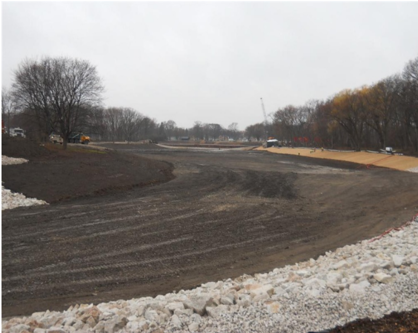
Zone 2A after completion of excavation and bank stabilization activities (11/26/2011)
