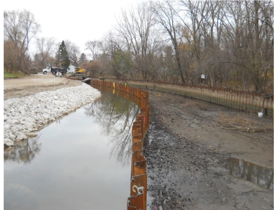
Zone 1 east dewatering and excavation (11/21/2011)
