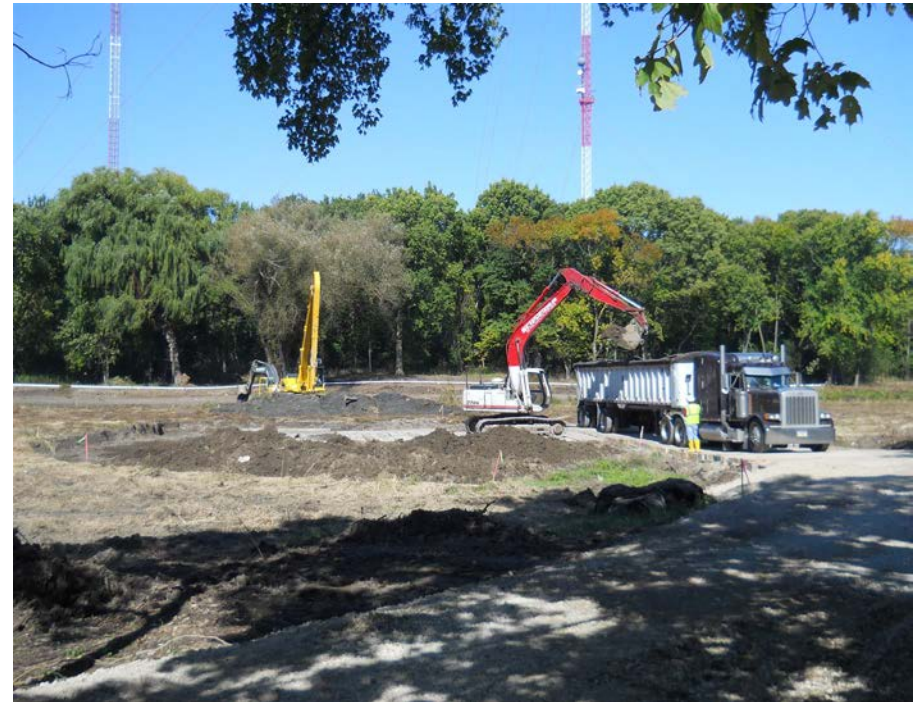
Excavation and hauling of TSCA material in Zone 2A
