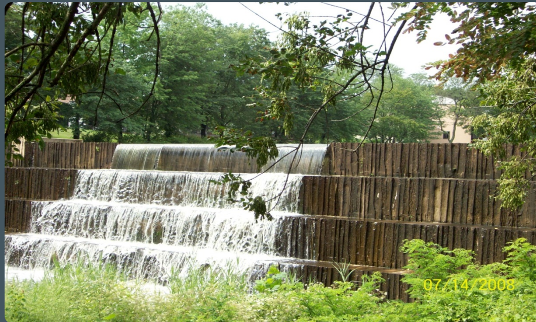
View of dam face (facing west)
