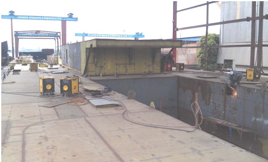
Pontoons Under Construction in Bangladesh
