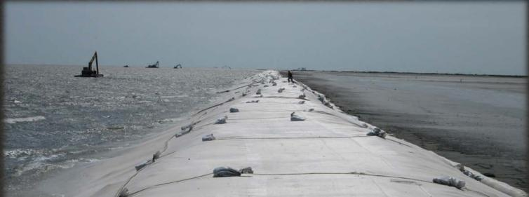
Installation of 4,620' of 50' wide scour apron over the reformed berm. Prior to placement of the apron the newly shaped berm was covered with 6 mil Visqueen. The apron was deployed and an anchor tube along each side was hydraulically filled to prevent the apron from being undermined by tide or surf.
