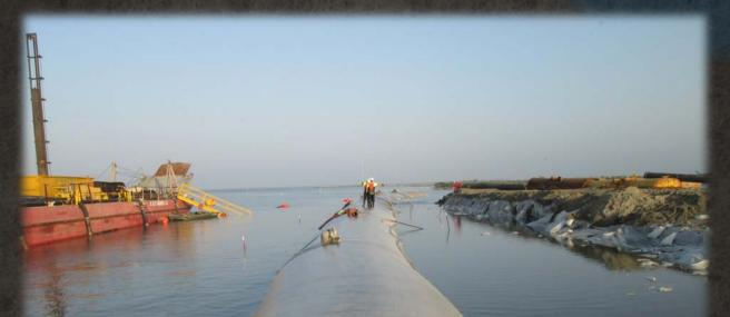
Installation of 400' of 30' circumference geotextile tubes, deployed and filled on top of 25' scour aprons with anchor tube on the sea side.
