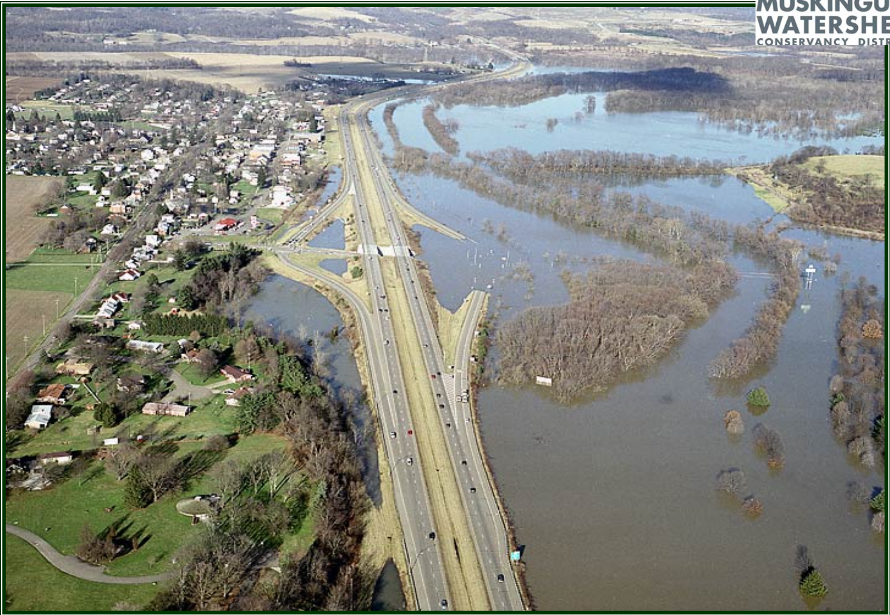
Looking North - Interstate 77 at Bolivar - January 2005
