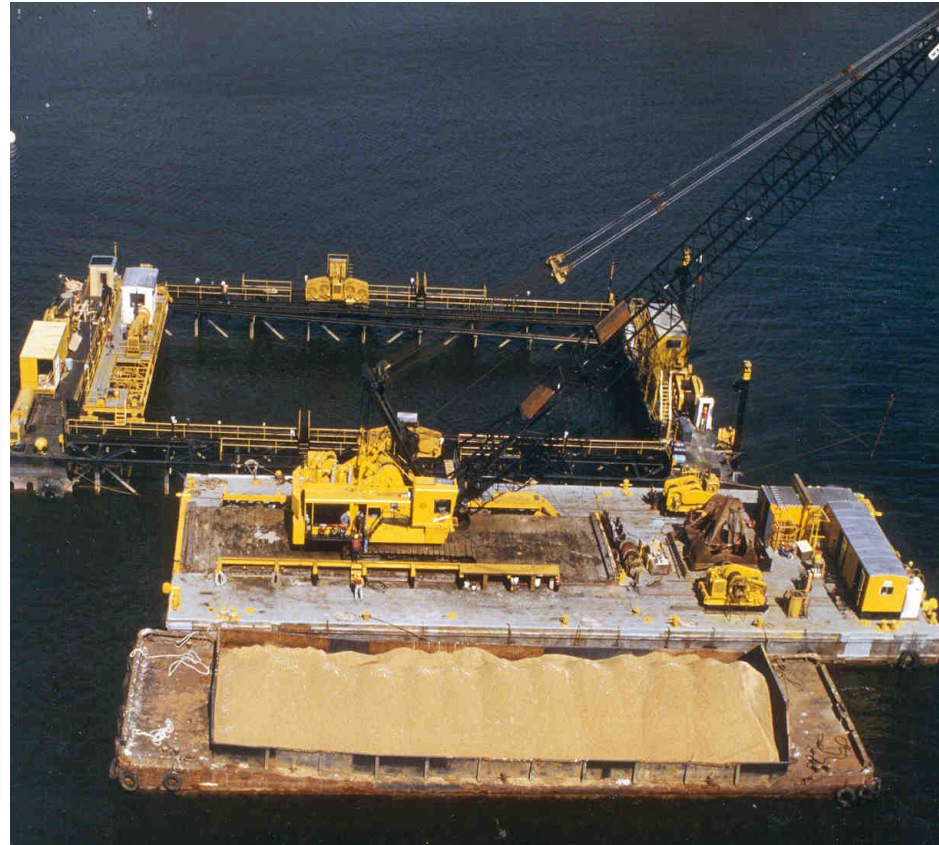
Fort McHenry Screeding Equipment
