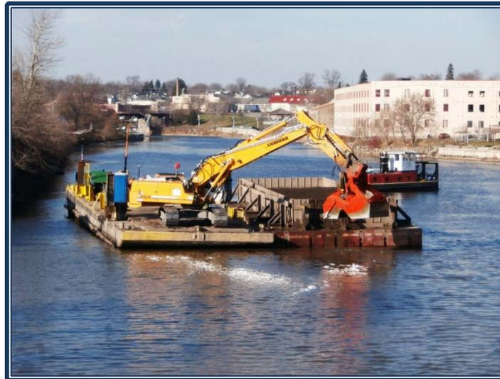
Figure 2 - Prototype environmental bucket designed for excavator use
