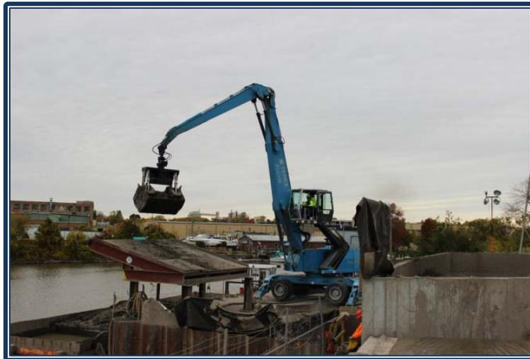
Figure 5 - Material handler offloading dredged sediment
