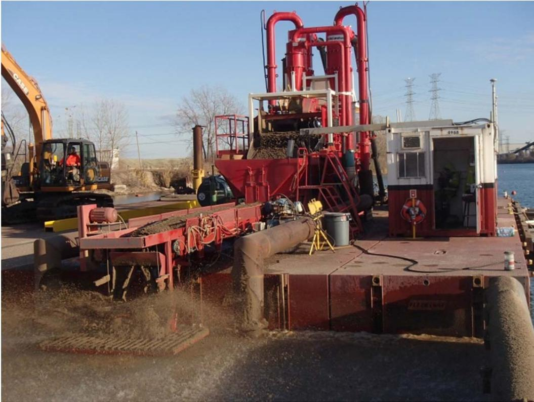
Figure 6. Broadcast capping system™ placing residual sand cover.
