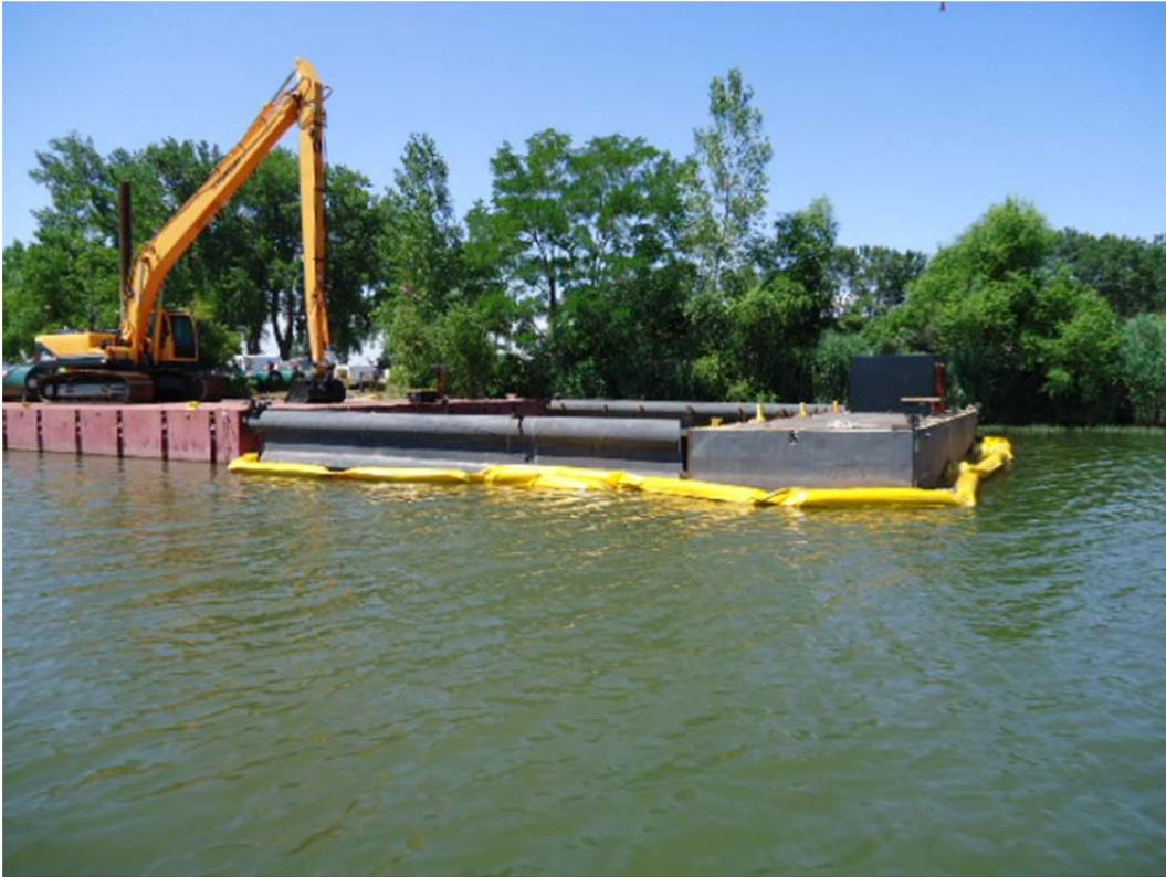
**Photo 2: Mechanical dredge removing TSCA sediment within silt curtain containment.**
