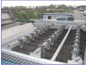
Figure 12. Water treatment facility.
