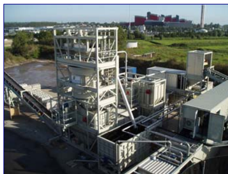
Figure 4. Mobile dredged sediment processing plant.
