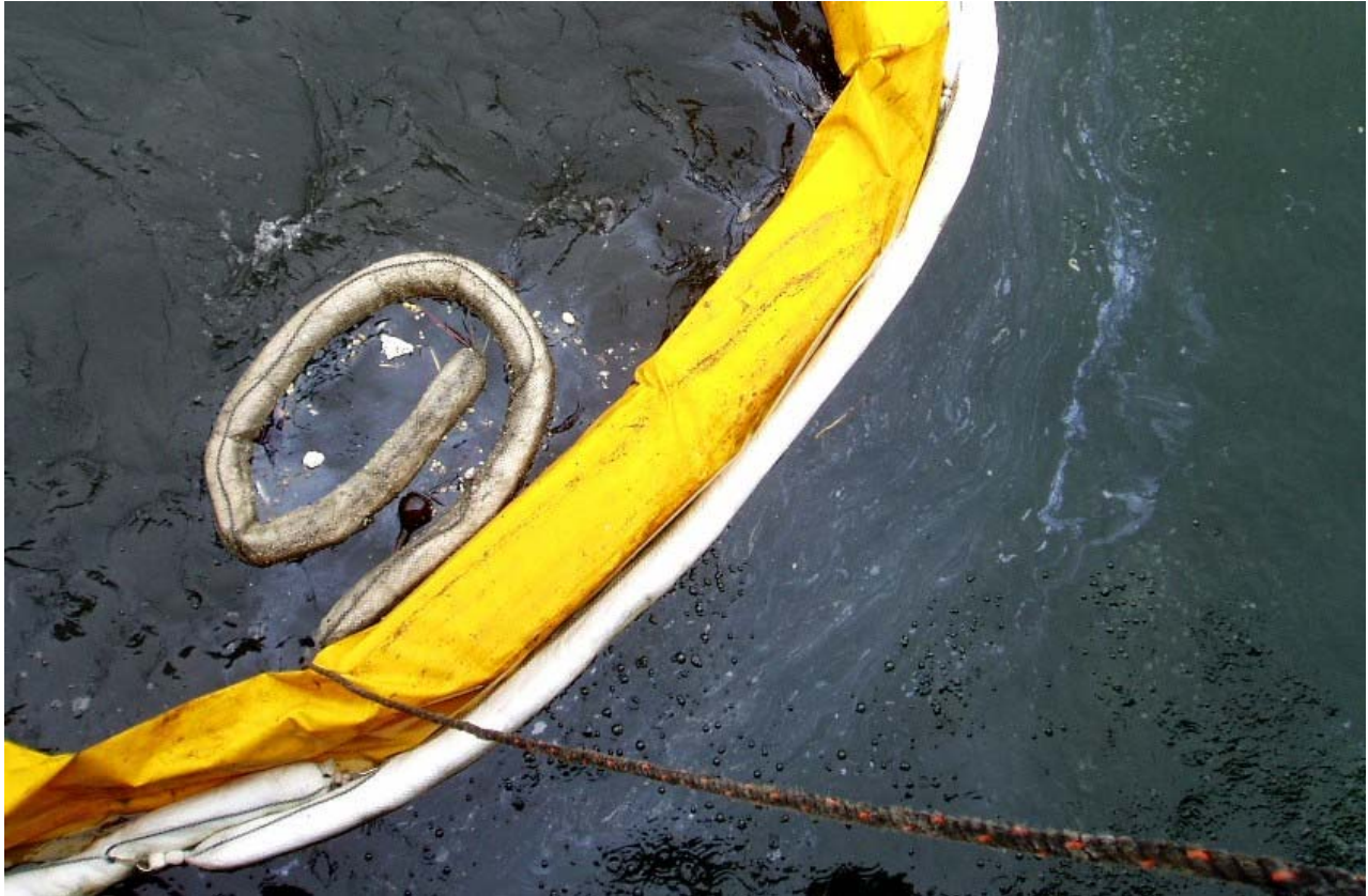
Figure 4: Creosote sheen rising from the sediments is contained by boom.
