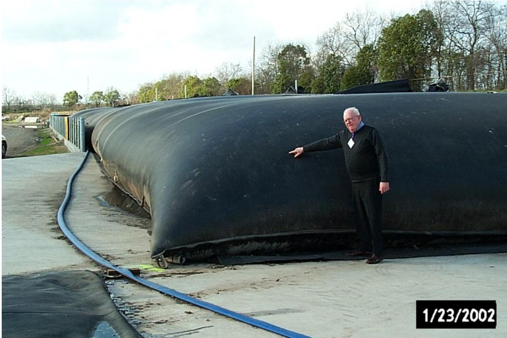
**Figure 15. Ninety foot circumference 270 ft long geotextile tube pumped with sludge to a height 7 ft**
