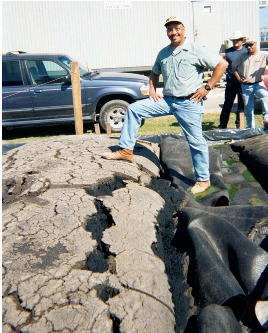
**Figure 12. Consistency of the sludge after dewatering and removal of the geotextile fabric top**
