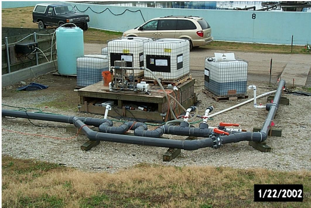
**Figure 10. Polymer feed system including valves and polymer tanks**
