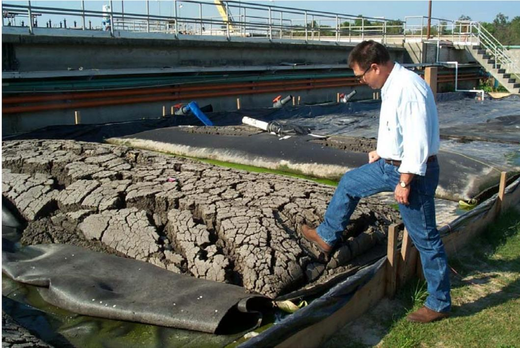
**Figure 13. Consistency of the sludge after one day of desiccation drying in the 4.5 m (15 ft) circumference tubes**
