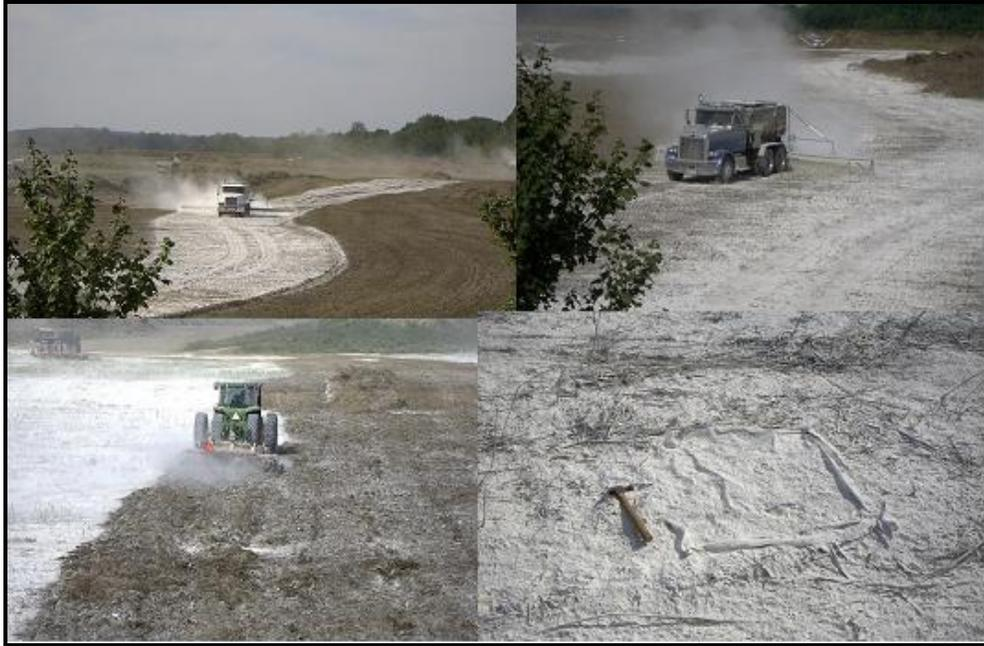
**Figure 4. Liming Operations at Courthouse Point CDF**
