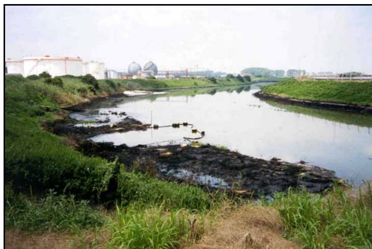
Figure14. Contaminated canal site.
