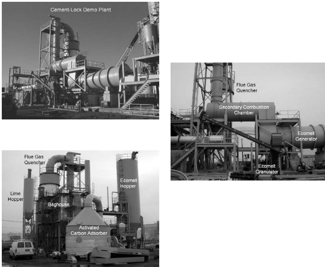
Figure 6. A general view of the Endesco thermo-chemical rotary kiln facility – Bayonne, NJ
