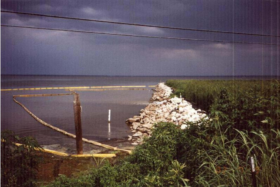
Figure 3. Dual curtain installation at Lake Palourde fill site.
