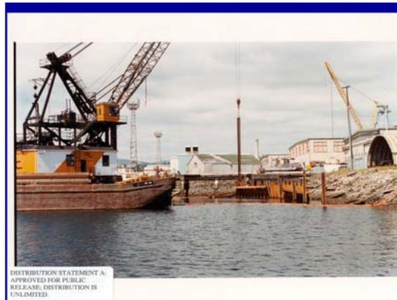
**Figure 8. Vertical cantilevered sheet piles.**
