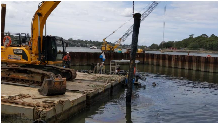
Removal of Old Piles with an Excavator
