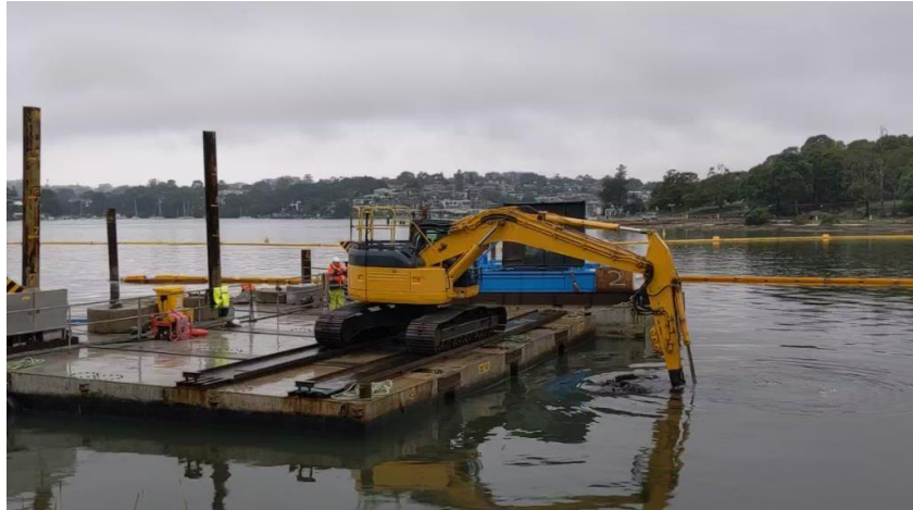
Access Dredge to Allow Barge Access to Shallow Areas
