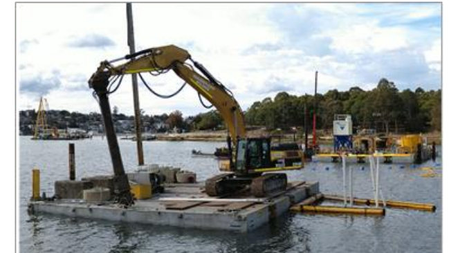
Mass mixing tool to build ISS raft
