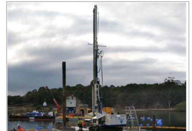
Auger mixing tool to build ISS columns
