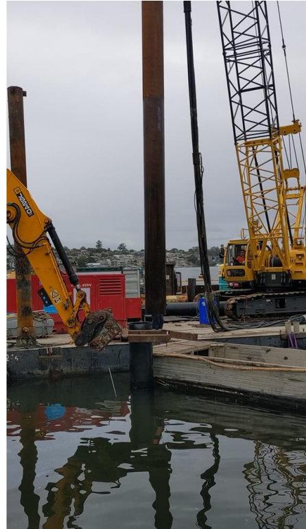
Removal of Old Piles with a Pile Driver
