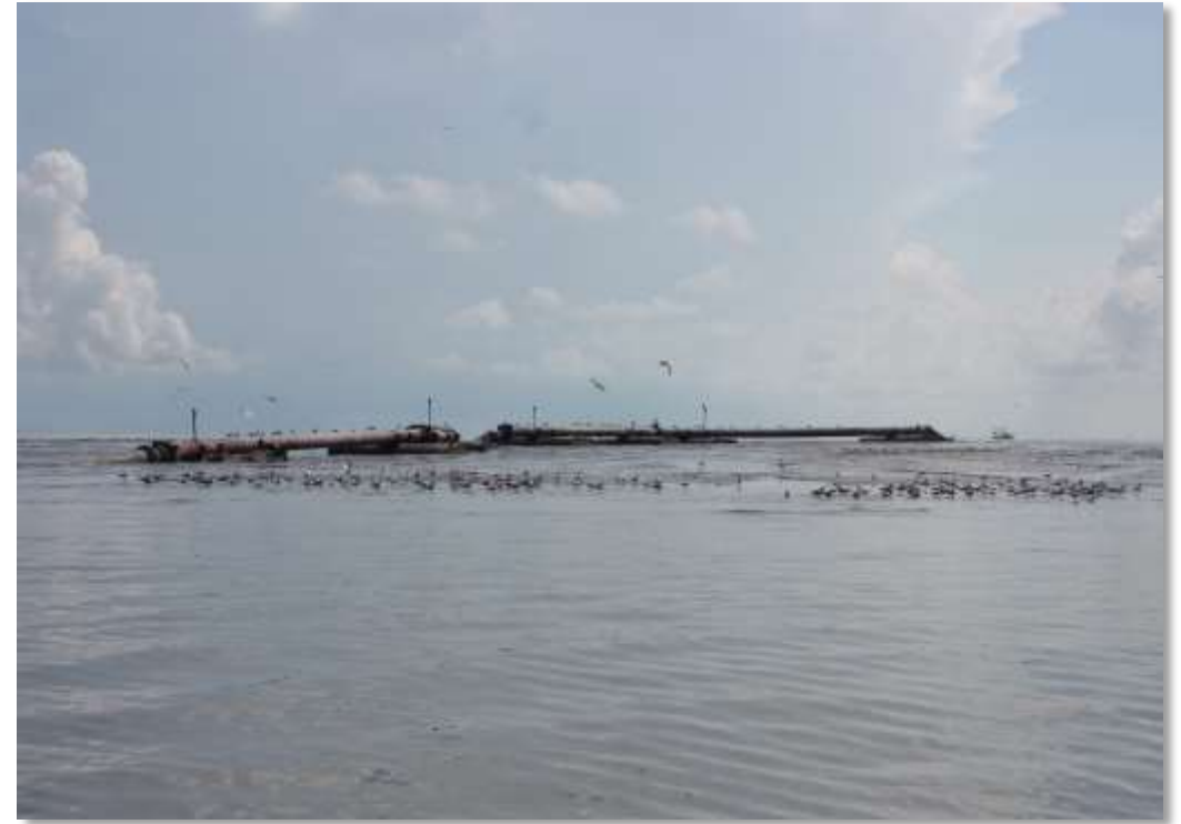
Gunn Island under construction in July 2016
