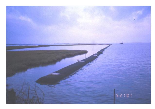
Top: 2,800 linear ft of geotube installed for restored marsh protection. Left: marsh mounds before and after being vegetated with *S. alterniflora*. Photo credit: Cherie O'Brian
