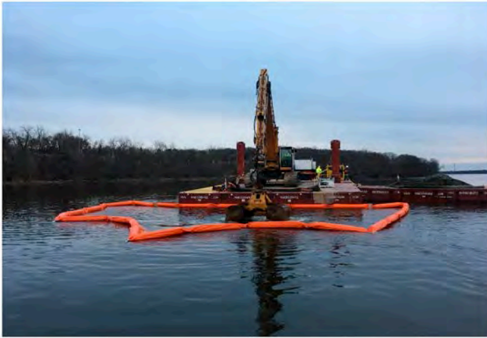
Placement Operations in PT9
