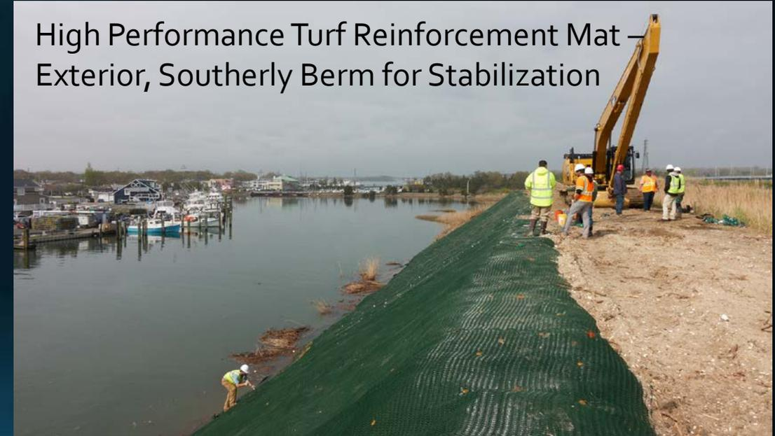
High Performance Turf Reinforcement Mat – Exterior, Southerly Berm for Stabilization
