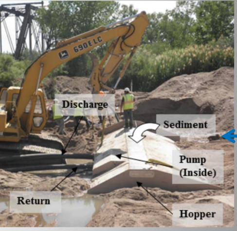
Grate Dimension: 9 m (30 ft) x 0.6 m (2 ft) Pump: 37 kW (50 hp) submersible
