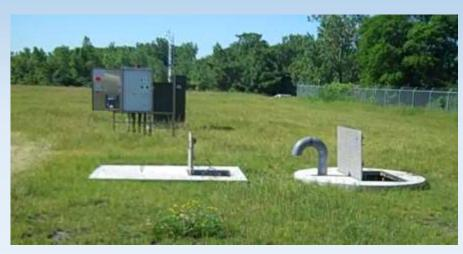
Lift Stations and Wells direct ground water back into the CDF
