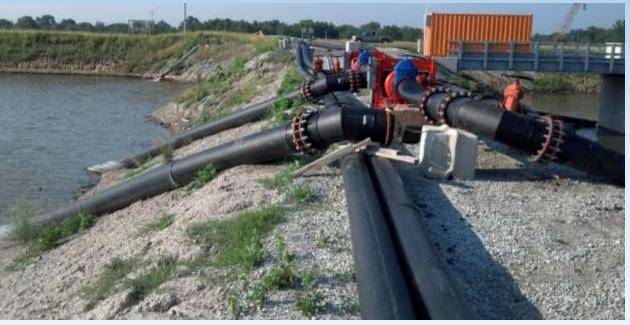
Water is also used in a manifold system to break up sediment placed on the debris screen to allow it's passage to the submersible pumps.
