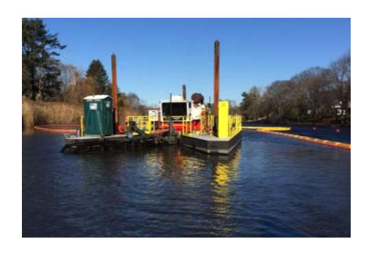
General Scope of Work – Contain hydraulic dredge site contaminated sediments within several work zones utilizing 3,400' of double walled TYPE 3 HD curtains to manage site turbidity
