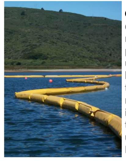
General Scope of Work – Contain construction sediments within each reservoir's work zones used to provide seismic and hydraulic upgrades at the three reservoirs built in 1888. Demolition, new tunnel liners, refurbishment or replacement of water management infrastructure with frequent barge traffic with turbidity managed utilizing 9,150' of tapered TYPE 3 **HD** turbidity curtains
