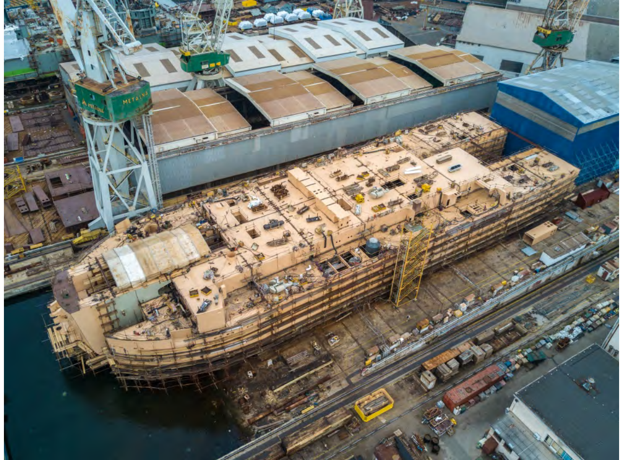
41 MW CSD under construction - Croatia
