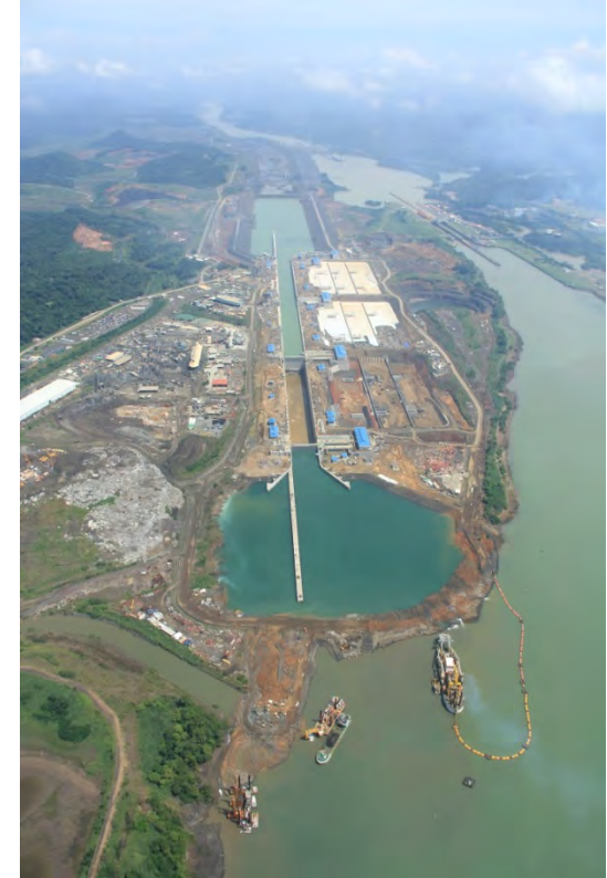
Panama Canal New Locks
