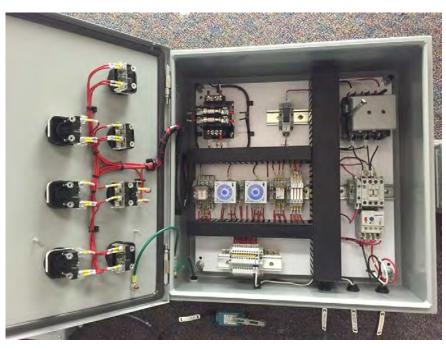
Our motor controller lab allows students to understand controller logic and operation through a mix of classroom and hands on training.
