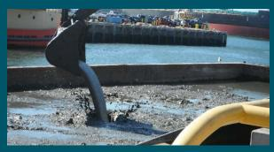
Stabilizing sediment with cement
