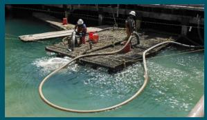
Sand placement using pneumatic pumping
