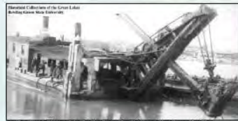
Scow-dredge No. 004, built in 1884 in the U.S. and abandoned in 1906. A similar vessel was located at the site. Photo taken late 1800s to early 1900s.
