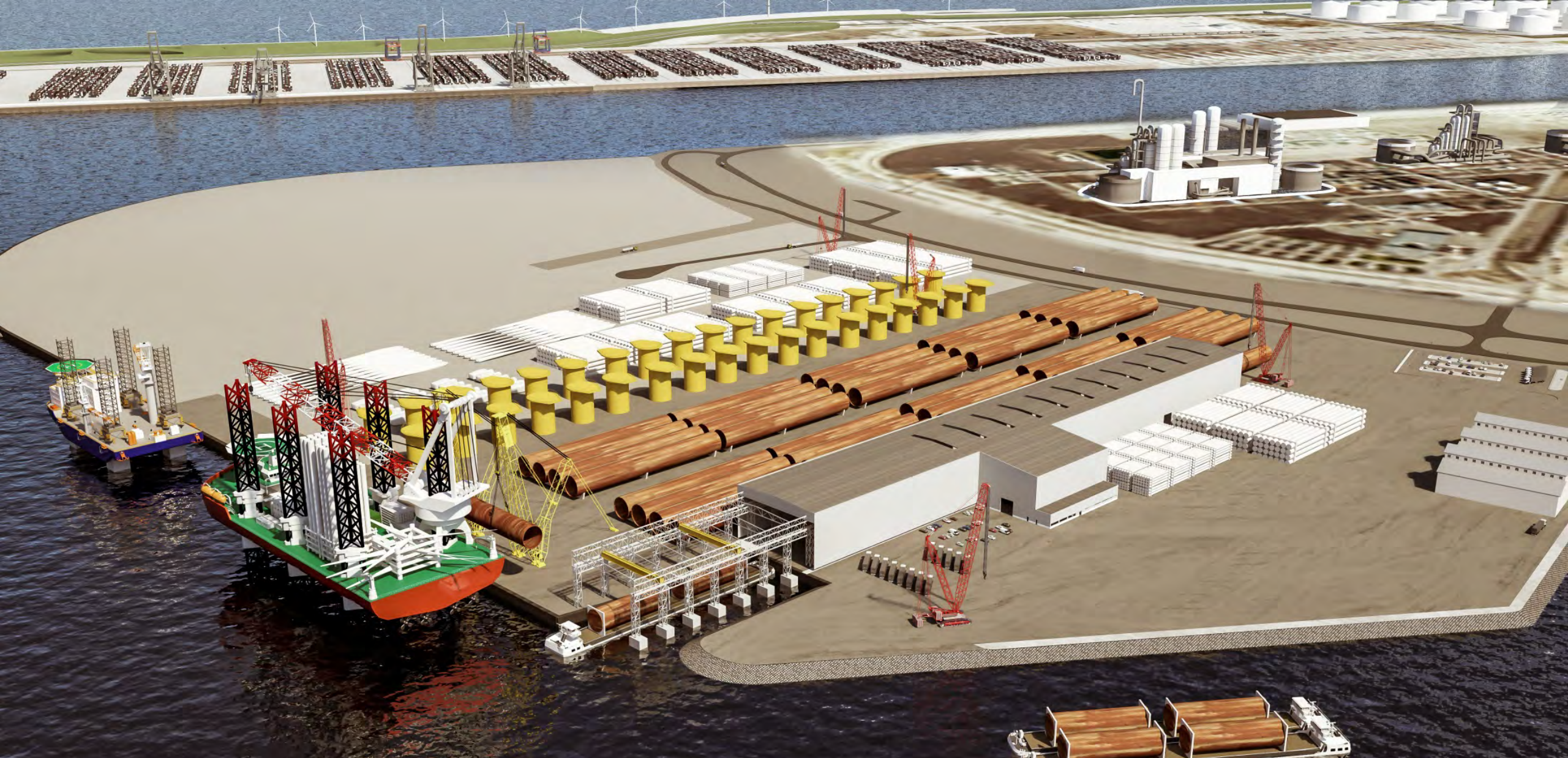
Offshore Terminal Rotterdam
