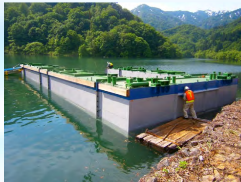
(Assemble of floating part)
