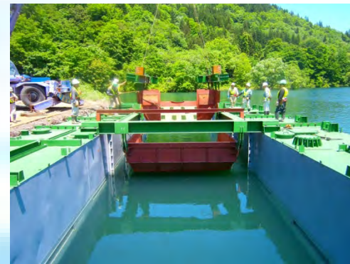
(Insert of Hopper part)
