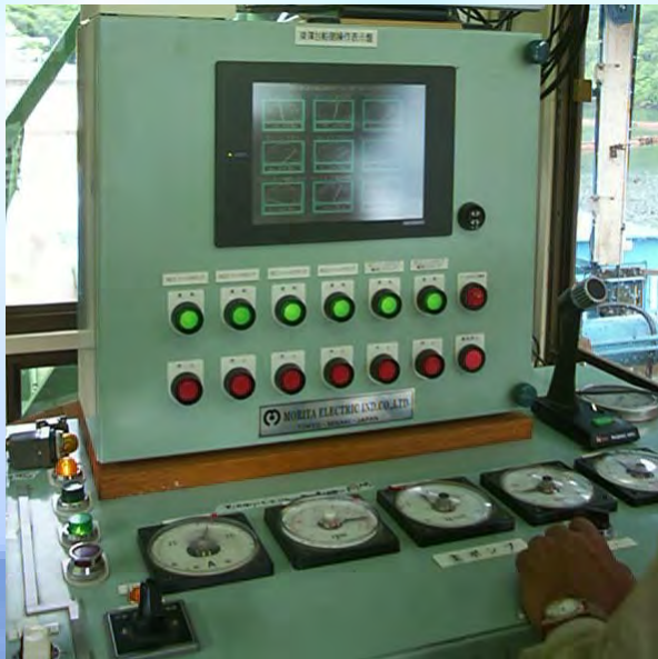
Remote control from Grab Dredger
