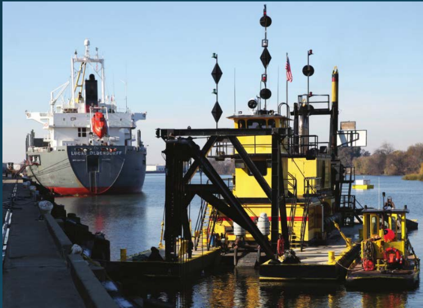
Hydraulic dredging at the Port of Stockton
