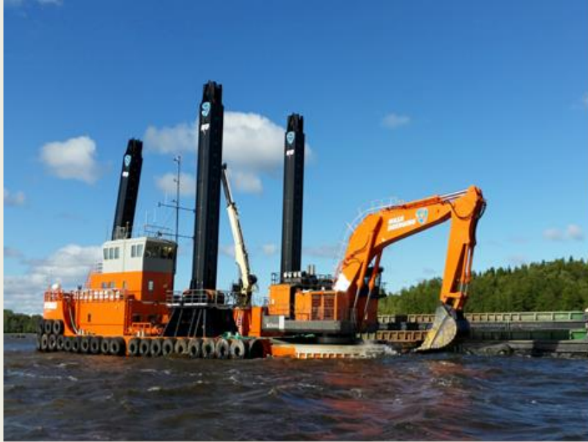
Hydraulic backhoe 'OPTIMUS' (Wasa Dredging Ltd.)
