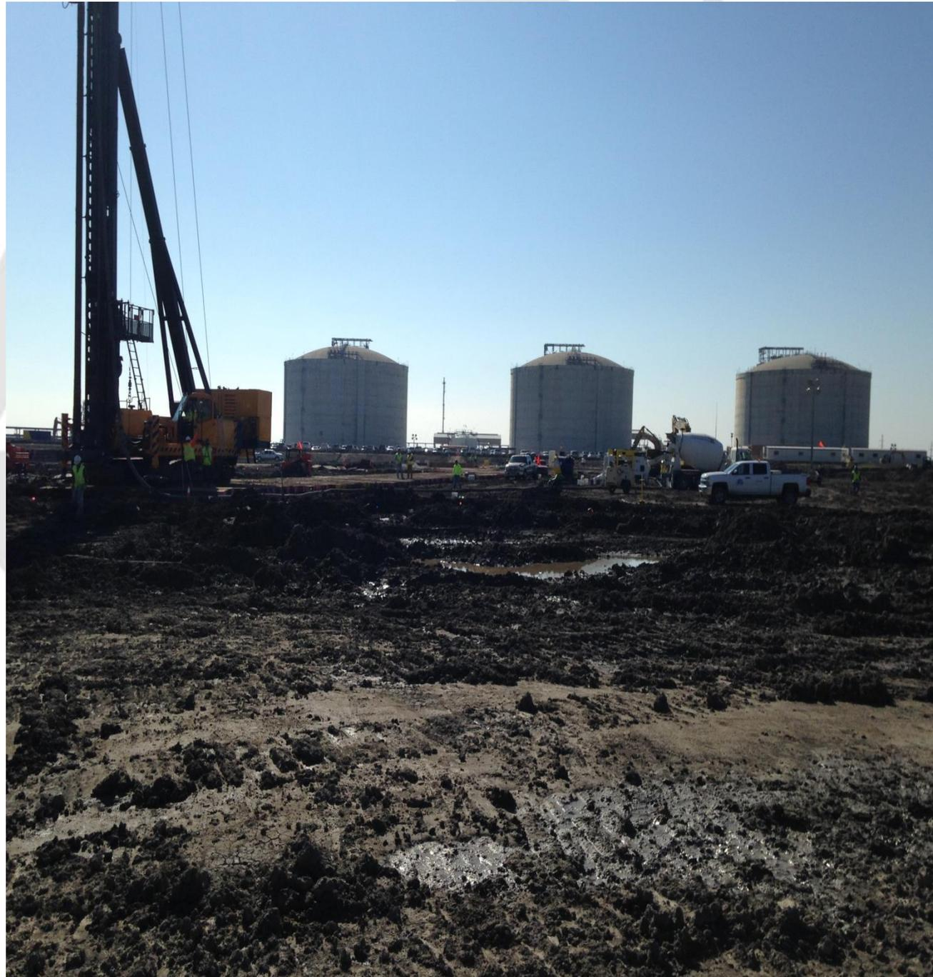
Soil subject to treatment. Soil has no bearing capacity. Wooden mat “roads” needed to move heavy equipment around on site
