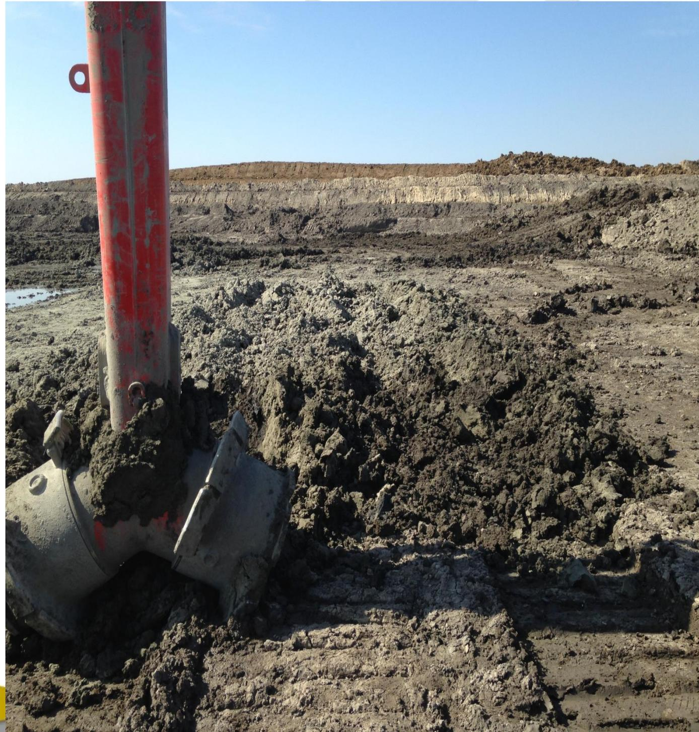
Test area after binder addition, PMX mixing, and compaction. Flagged for sampling and testing.
