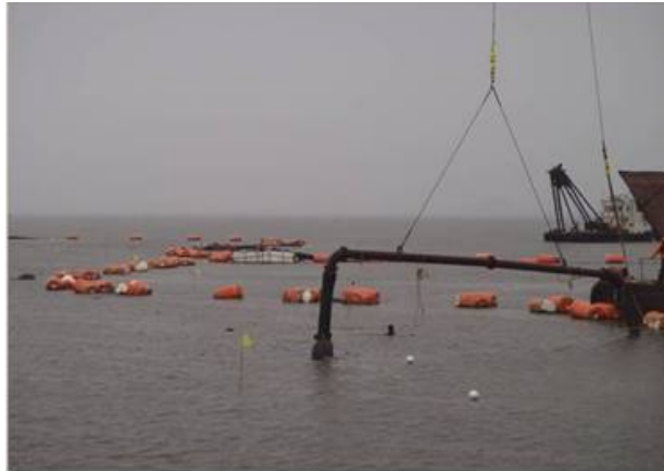
Start of geotextile tube filling
