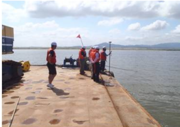
Setting out using GPS
