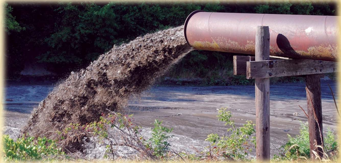
Dredge designed to pump on existing pipeline system
