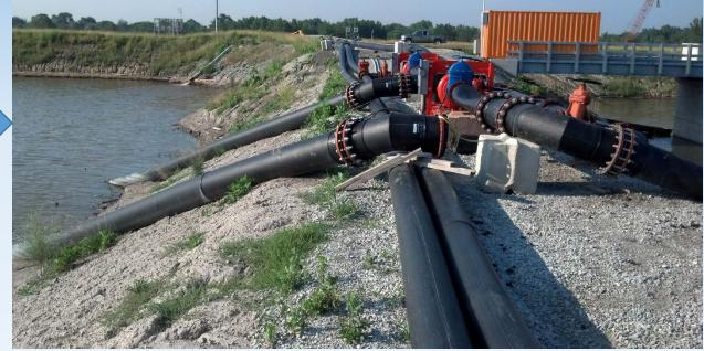
Water is also used in a manifold system to break up sediment placed on the debris screen to allow it's passage to the submersible pumps.
