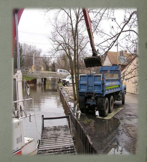
Direct loading is when an excavator will excavate the material directly from the channel and put it right into a truck Barge loading is the method using amphibious excavator loading a hopper barge and pushing the barge to a dedicated load out site.
