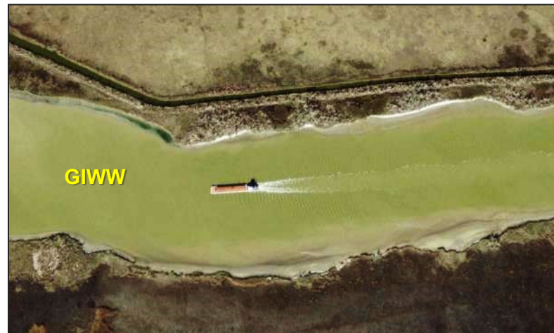
GIWW Bank Erosion
