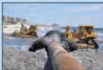
Slurry of sand being pumped onto the beach and moved to the berm
