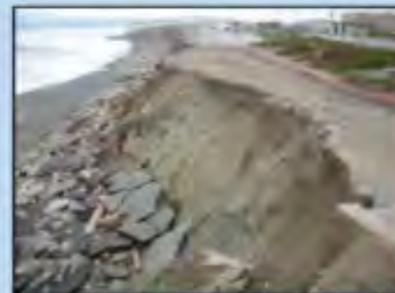
Wave caused bluff failure South of Sloat Boulevard
