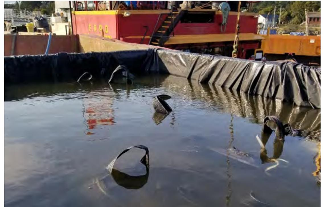
GAC supersacks were soaked in watertight containers on mixing barge and agitated to remove entrained air (24 hrs)
