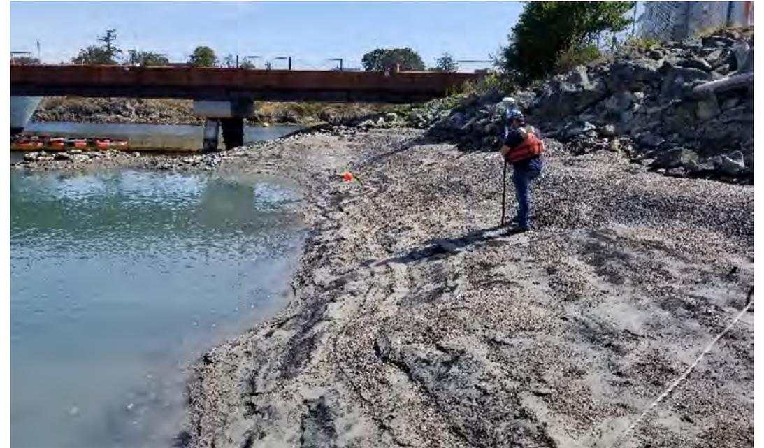
Daily/nightly progress surveying and engineering review to confirm areas and minimum thicknesses of multiple cap layers
