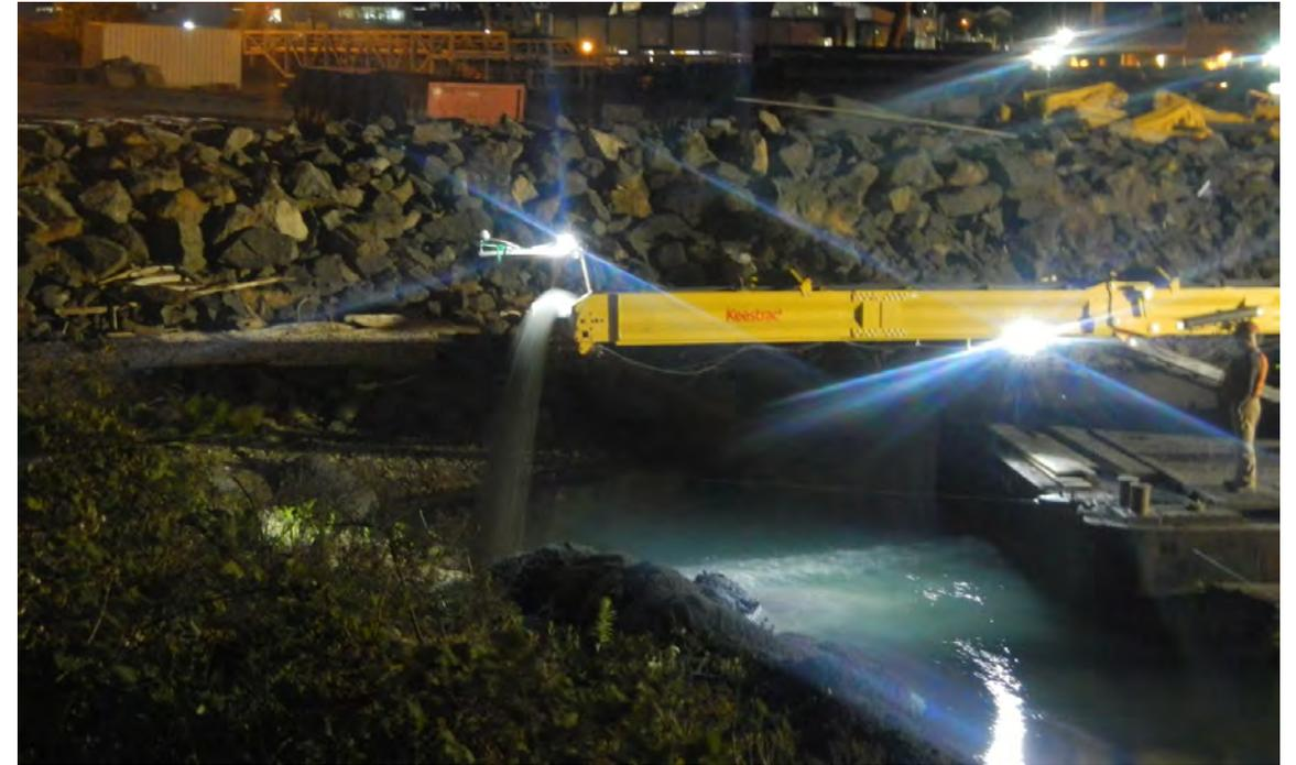
Conveyor mounted on low draft/maneuverable barge for restricted access placement due to shallow water and working tides
