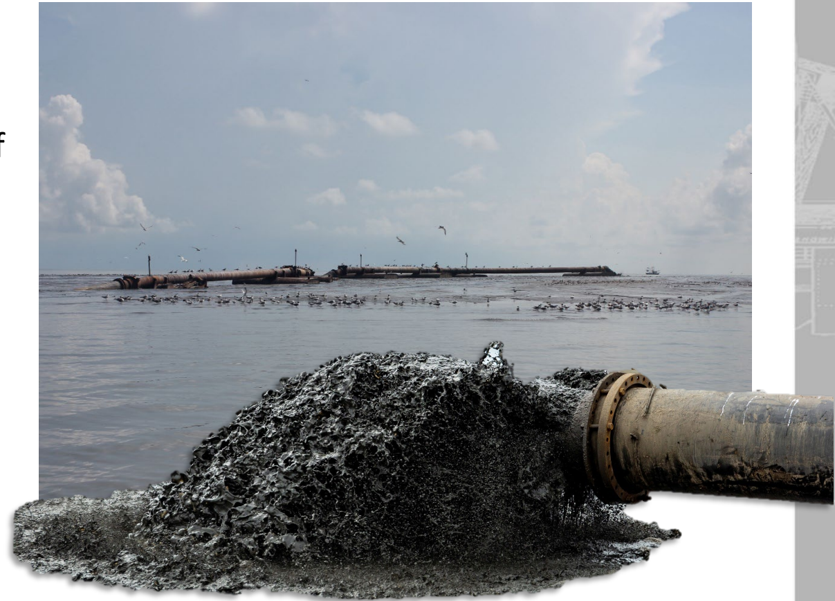
Pipeline transporting dredged sediment to Gunn Island in July 2016.
