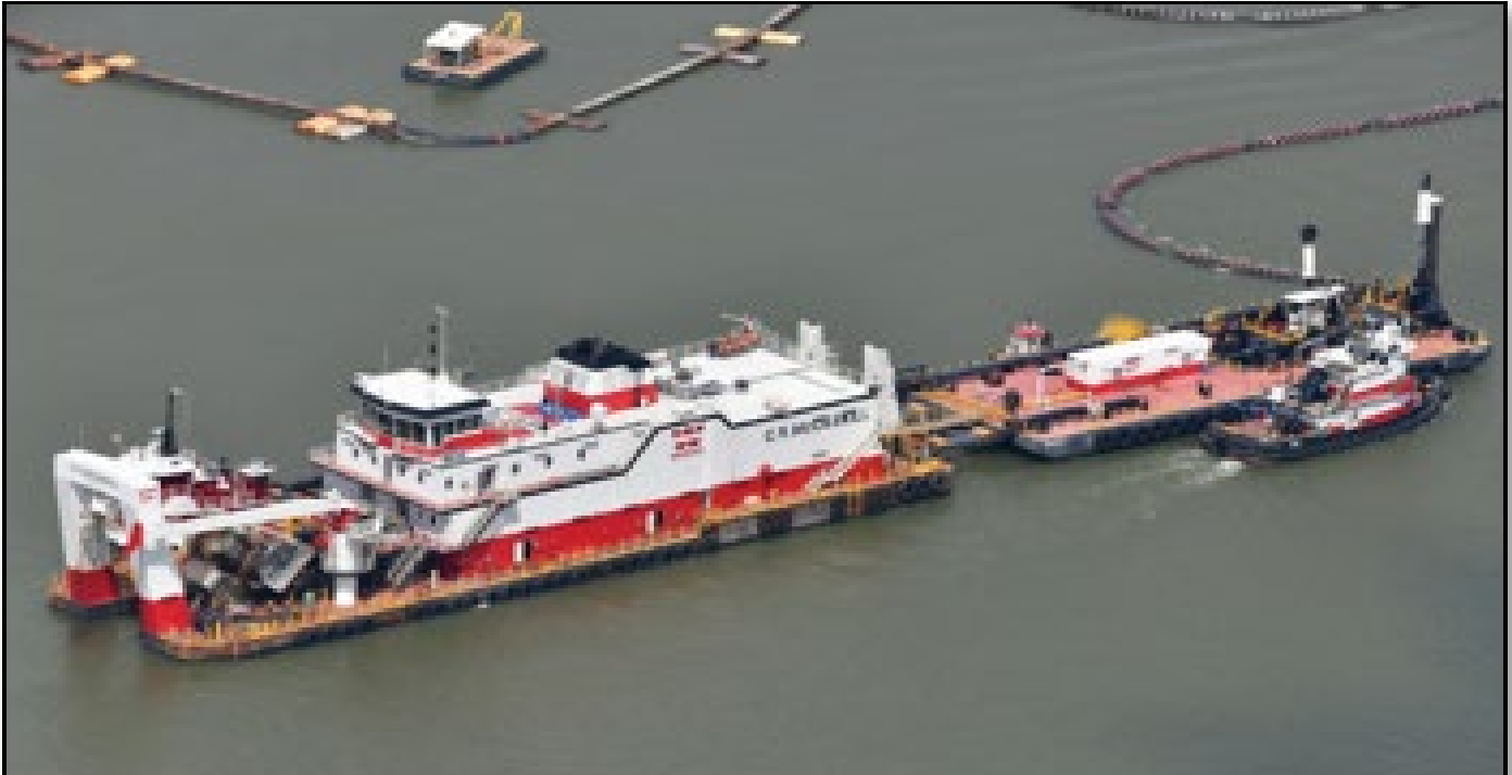
ONGOING. Redfish to Bayport 8.2 MCY Three Bird Island Marsh
