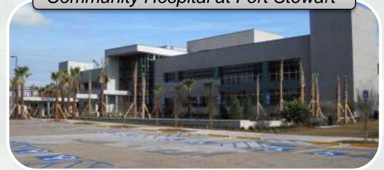
Community Hospital at Fort Stewart
