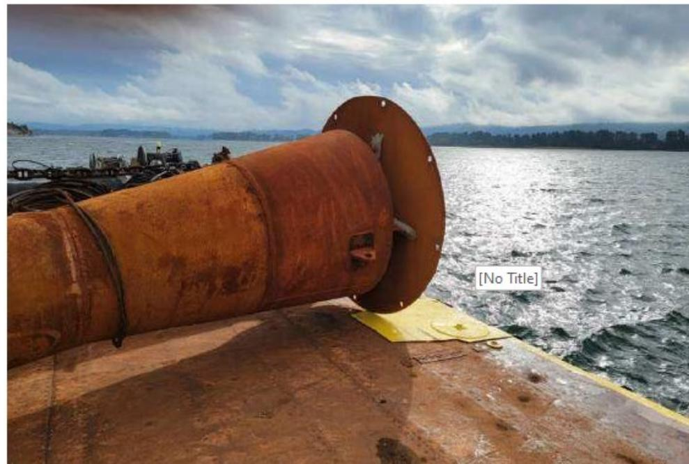
Diffuser in final stage of fabrication, MAR 2021
