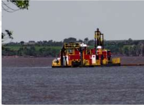
4 PORTABLE CUTTER SUCTION DREDGES
