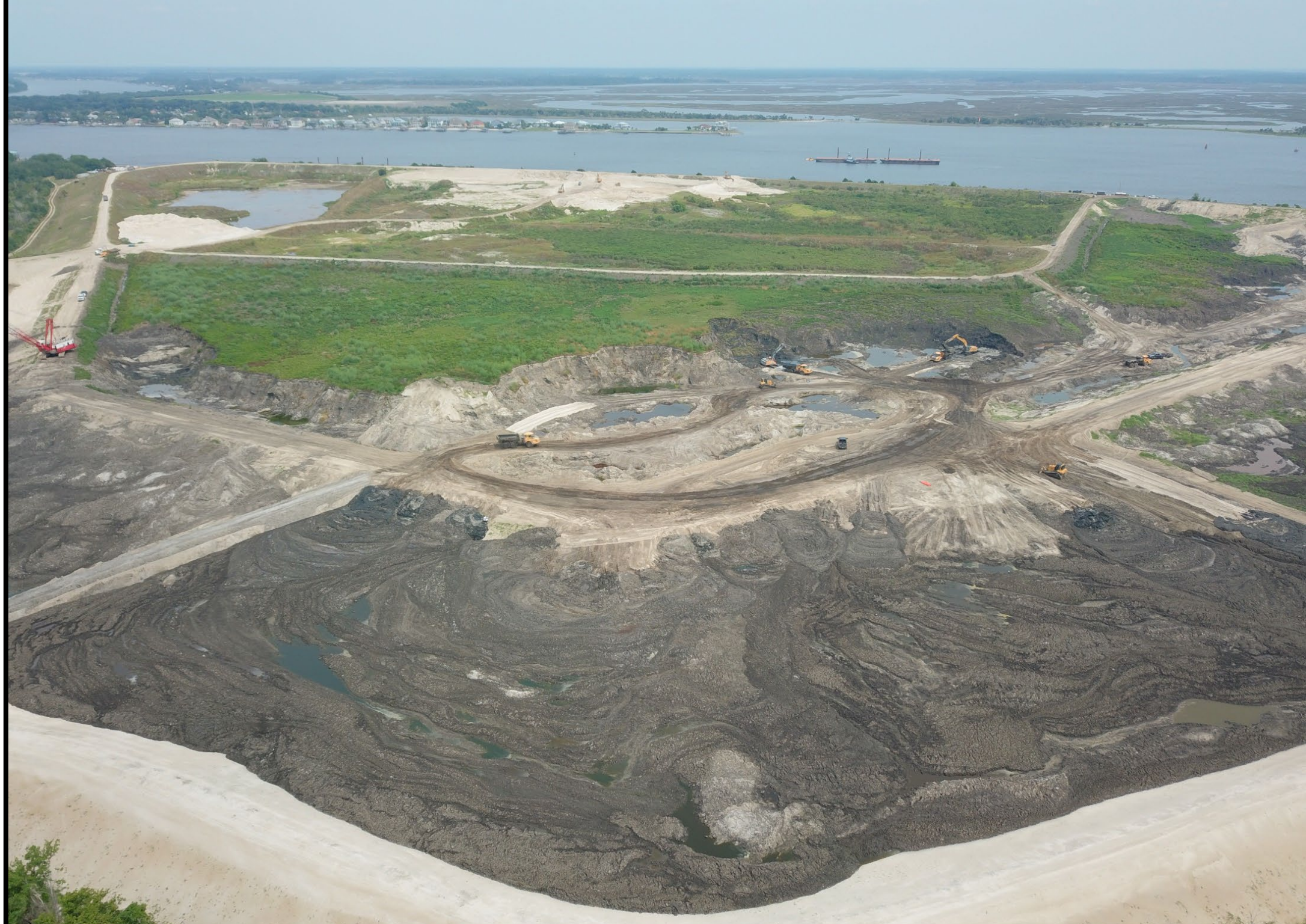
Buck Island Cell B – Temporary cross dike wall to contain material
