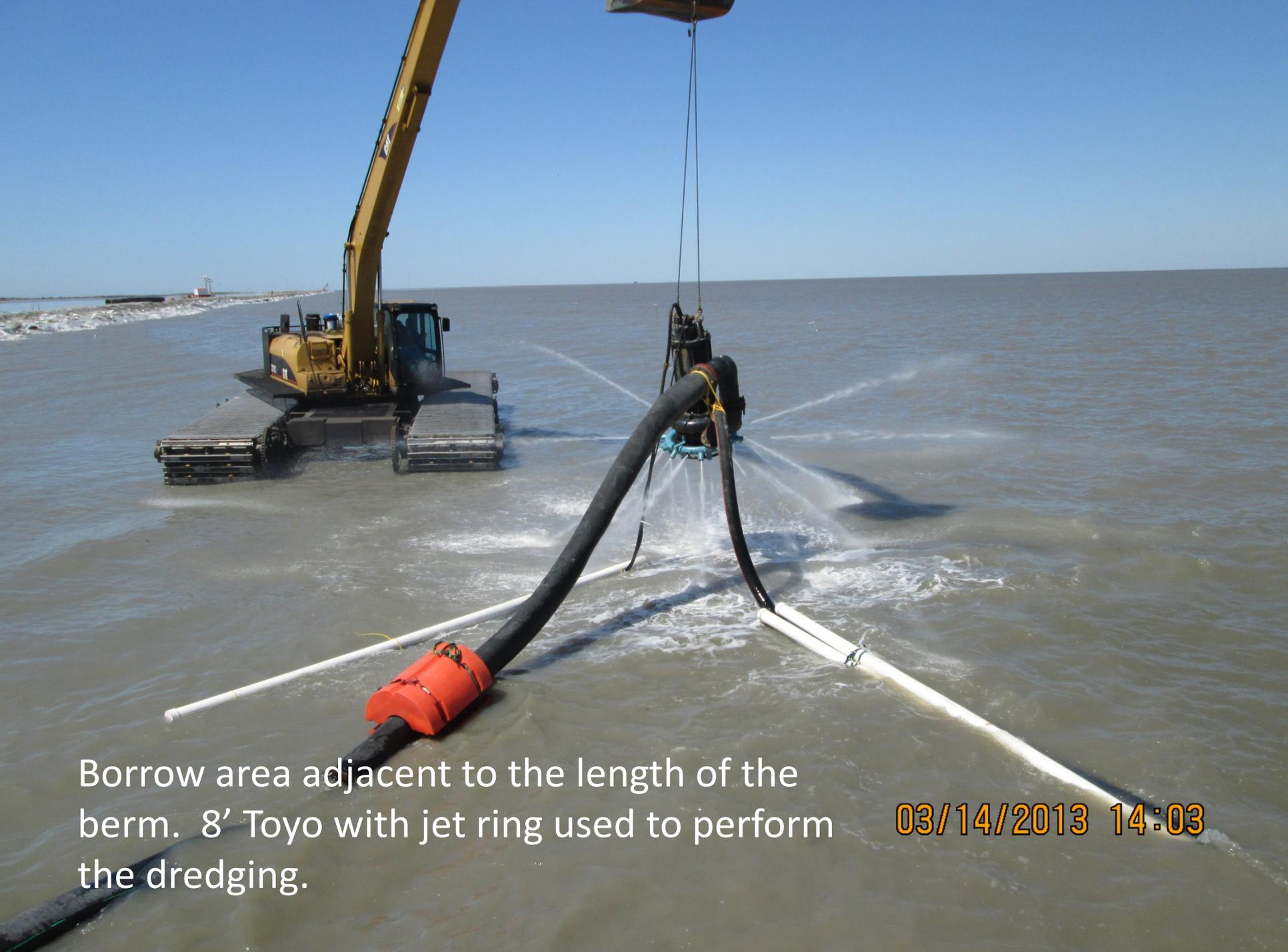
Borrow area adjacent to the length of the berm. 8' Toyo with jet ring used to perform the dredging.
