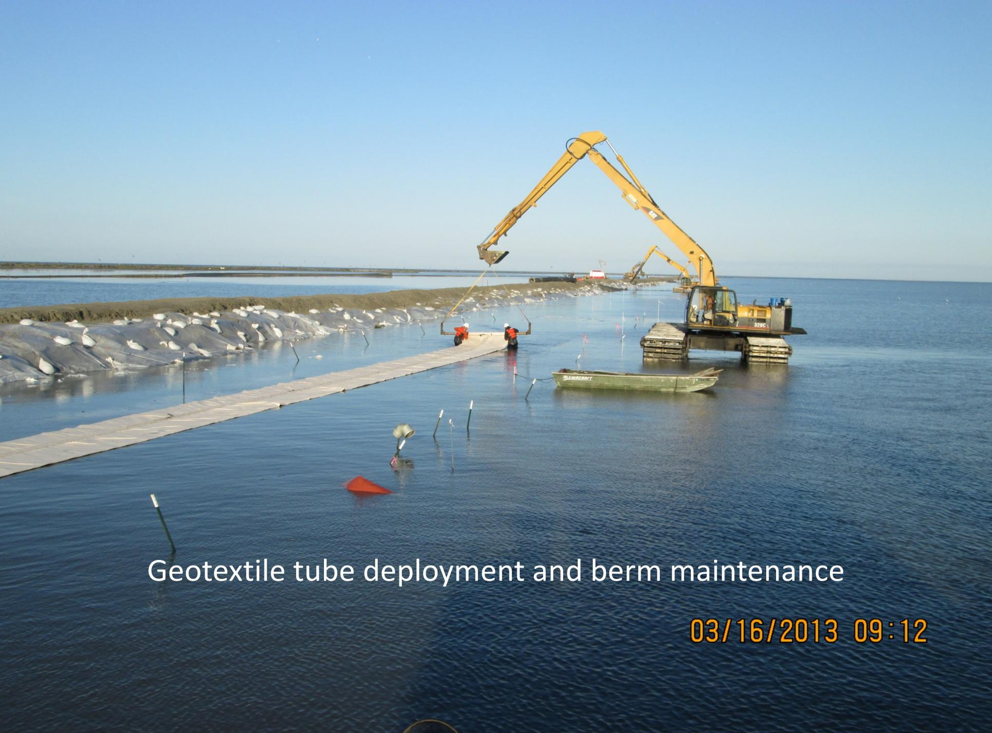
Geotextile tube deployment and berm maintenance
