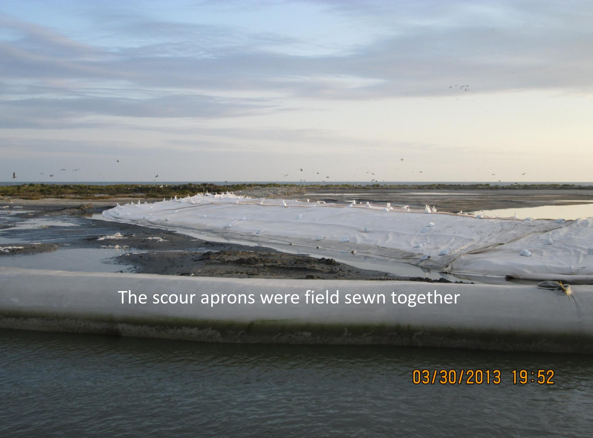
A wide-angle photograph of a coastal area during sunset or sunrise. A large, white, rectangular scour apron is laid out on a flat, dark surface, possibly a beach or a tidal flat. The apron is held in place by numerous white sandbags or weights. The apron is field sewn together, with visible seams and a yellow rope tied to a corner. In the background, there is a line of green vegetation and a body of water. The sky is filled with many birds in flight, and the overall lighting is soft and golden.
