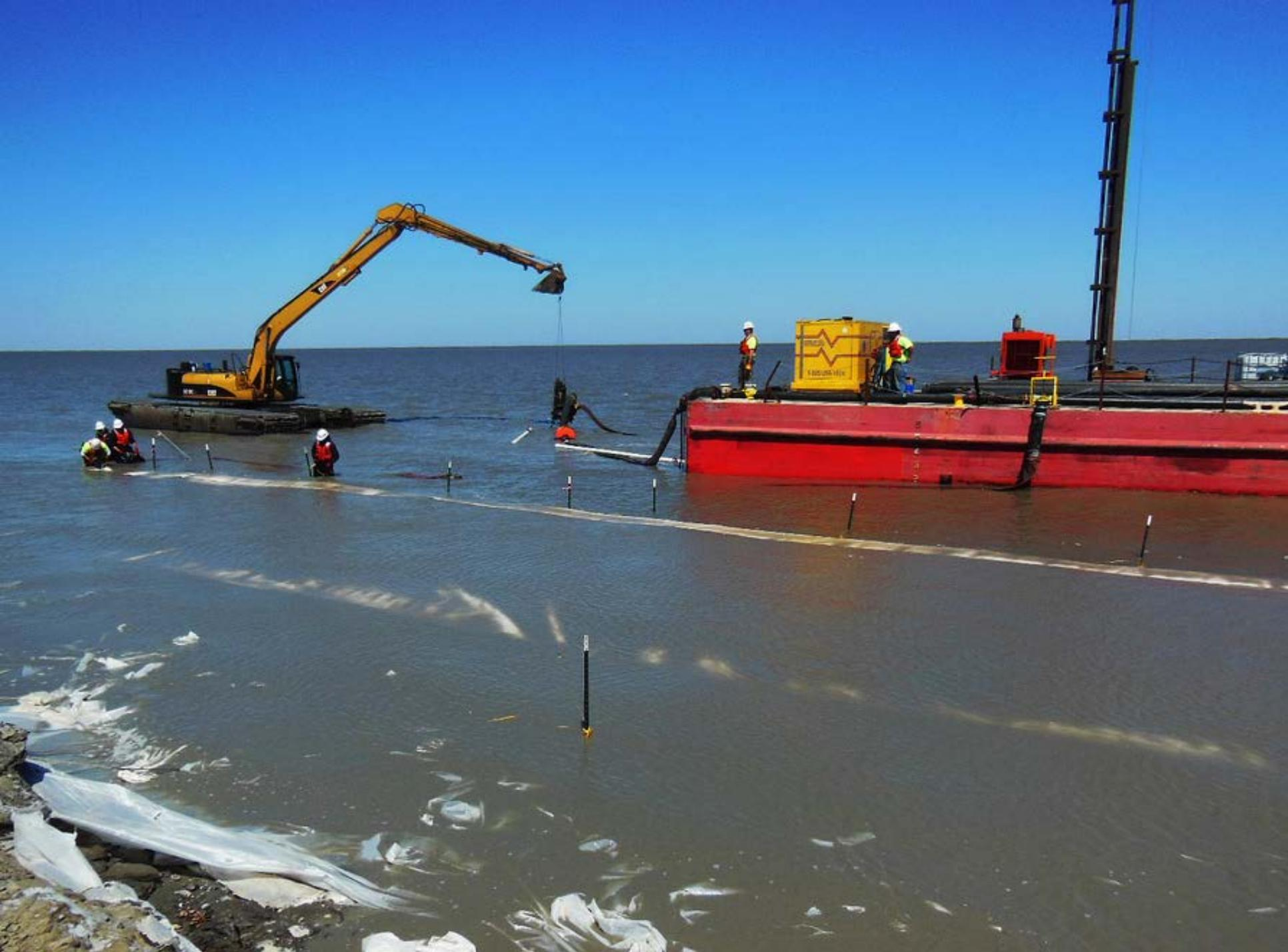
Geotextile tubes being filled
